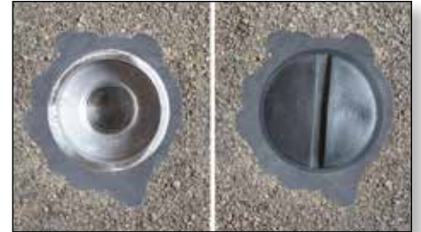
The anchor cup securely installed shown with and without plug cap
